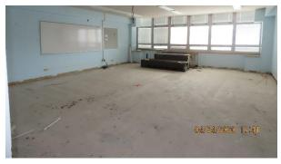
If the existing concrete does not have a vapor barrier we need to install a MRB (Moisture Reduction Barrier) on the concrete prior to the floor installation.
