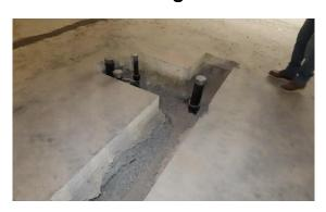
We should plan on performing a test core or review the plumbing trenches as soon as possible, to verify the presence of a vapor barrier.
